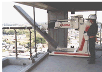
Figure 3 The KAJIMA “Mighty Hand” panel-holding construction robot.
